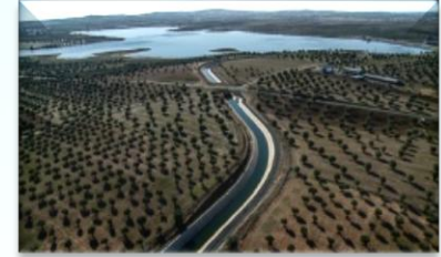
General Irrigation System
