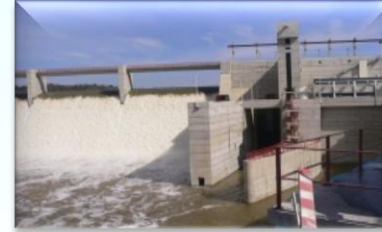
Pedrógão Mini Hydroelectric Plant
