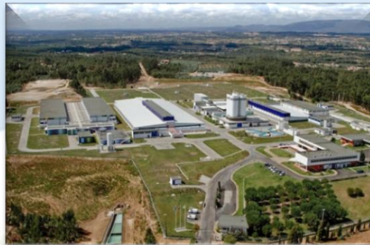
Asseiceira Water Treatment Plant
