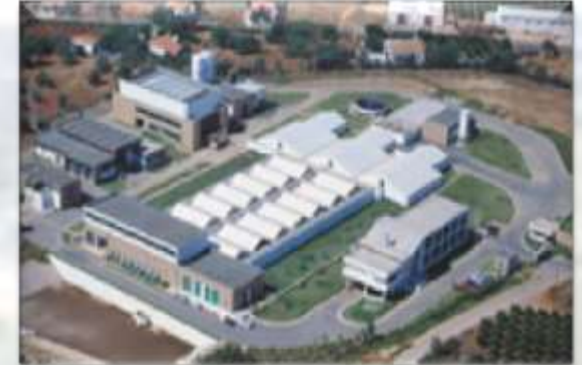
Alcantarilha Water Treatment Plant
