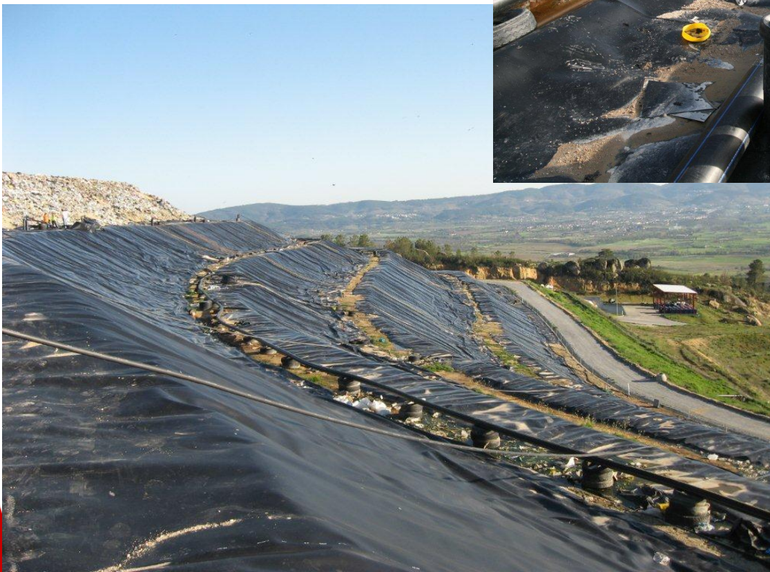
VALE DO LIMA LANDFILL - Portugal Biogás Collect with Energy Valorization 2000 kW
