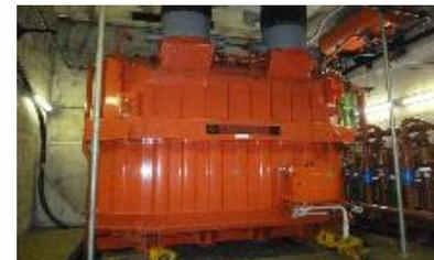
Scope: 160 MVA transformers maintenance, with replacement of coils
