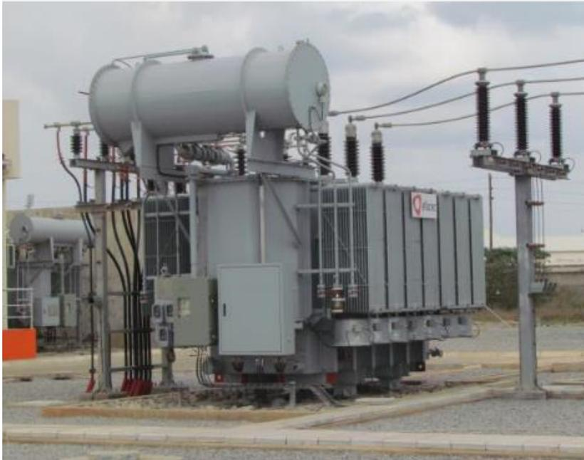
Core Type 40 MVA, 66 / 33 kV Transformer
