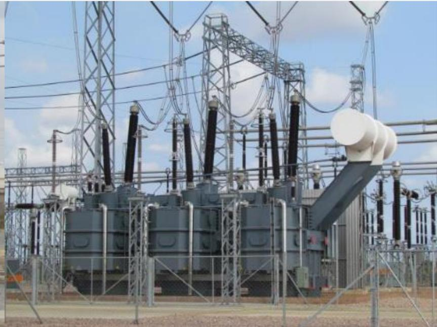
Shell Type 400 MVA, 400 / 275 / 11 kV
