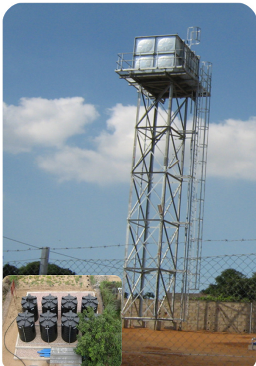
16 Small Systems Constructed in Maputo Peri-Urban areas
