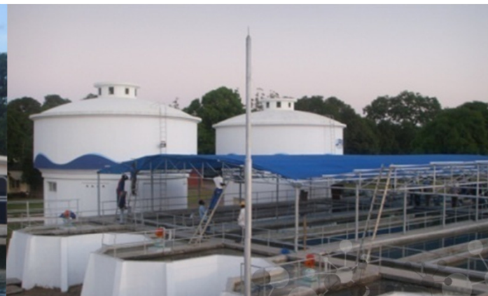
WTP - Beira (Cap.: 60,000 m 3 /day)
