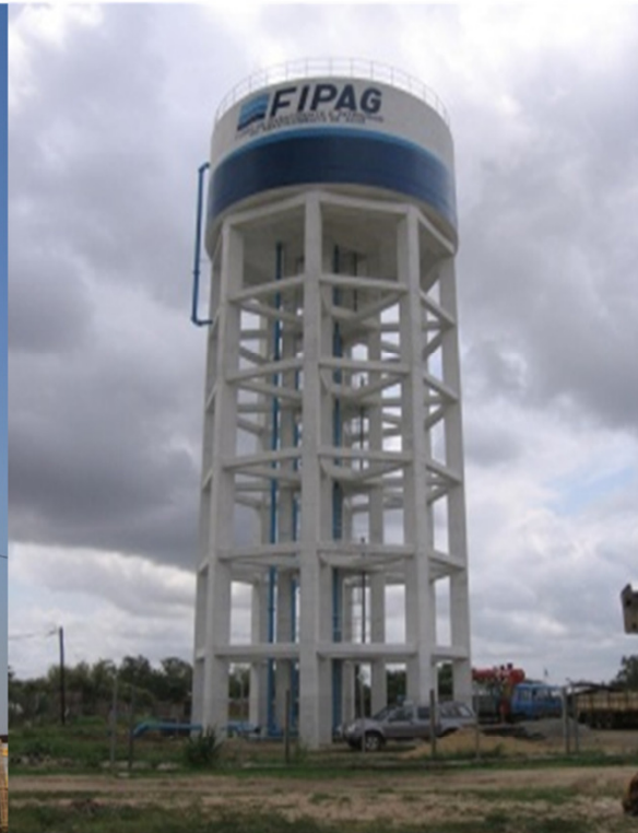
Reservoir/Distribution Water Tower - CHÓKWÊ
