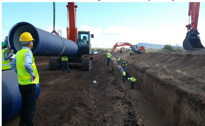
Pipe Storage in Moamba
