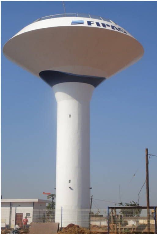
Distribution Water Tower - CHIMOIO
