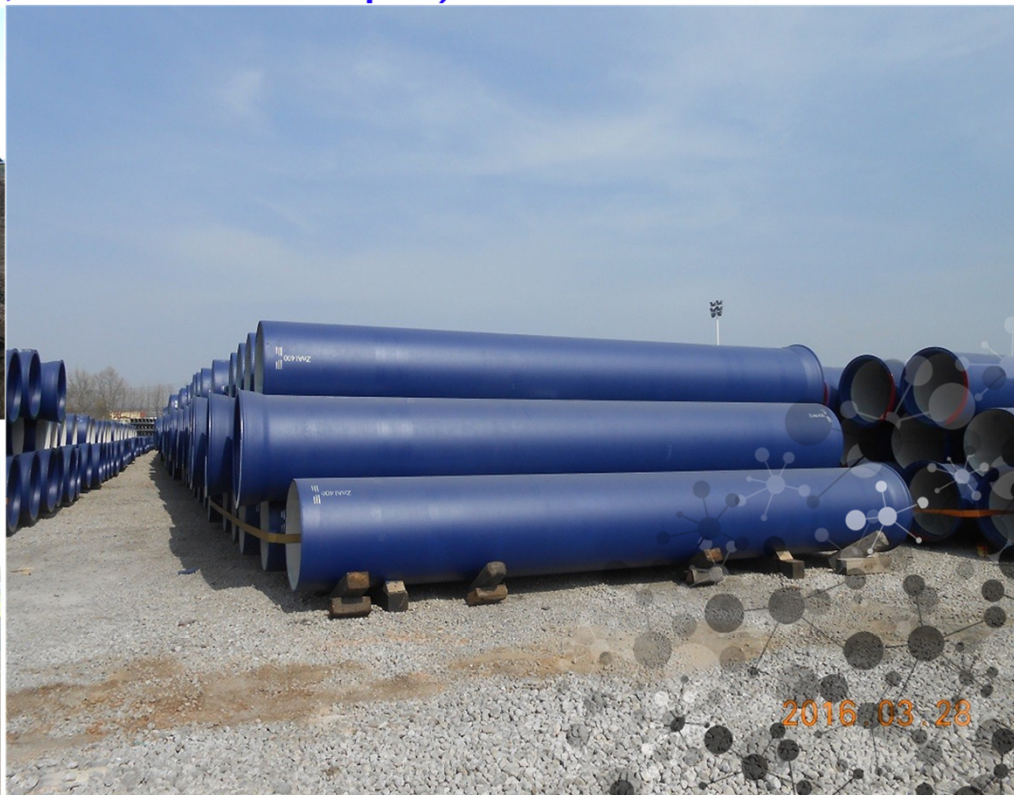
Pipe Storage in Moamba
