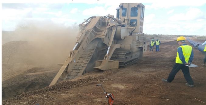
Excavation with Trencher M5
