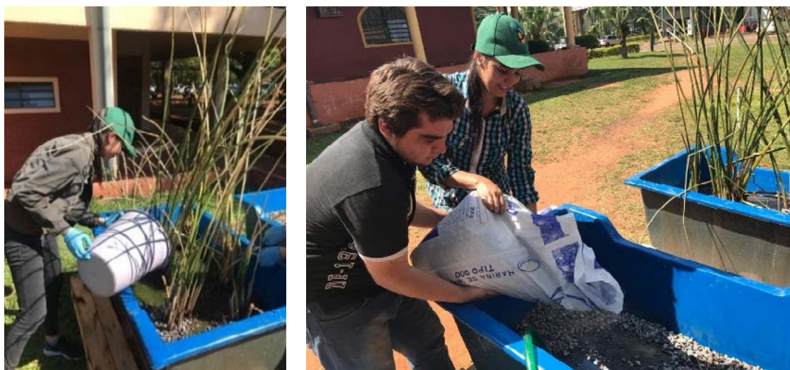
Figure 1. Set and started up of the pilot scale wetlands HA y HC
