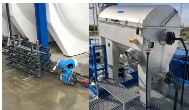
Figure 1. The figure shows the concentrator system composed of the flocculation tube (left) and the rotary drum sieve (right).
