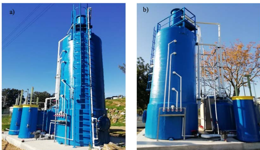
Figure 2. Photos of the UASB PUSH® prototypes installed at the Lagos (a) and Loulé (b) WWTP
