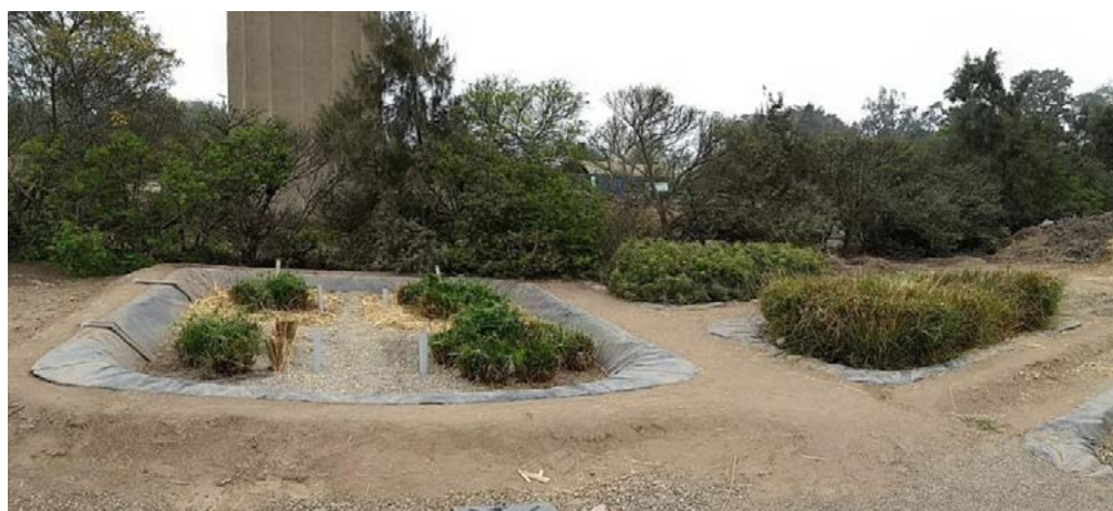
Figure 1. French System of UNALM. Left: 1 st stage (French cell); Right: 2 nd stage (vertical flow subsurface wetlands)
