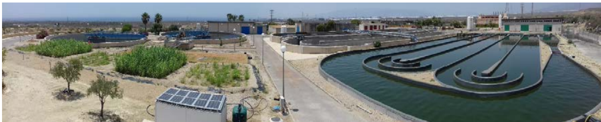
Figure 2. Panoramic view of El Toyo WWTP with the experimental demo plant (raceway and wetlands)
