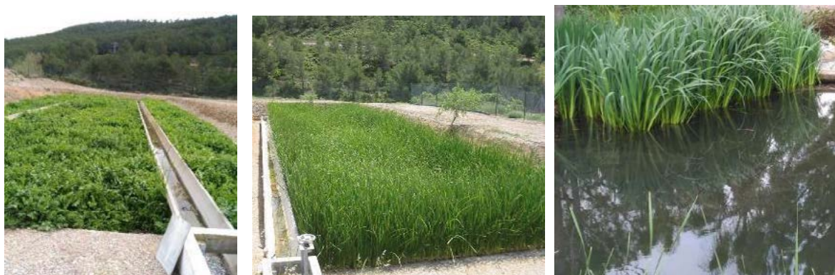
Figure 1. Photographs of the studied subsurface and surface flow CWs.
